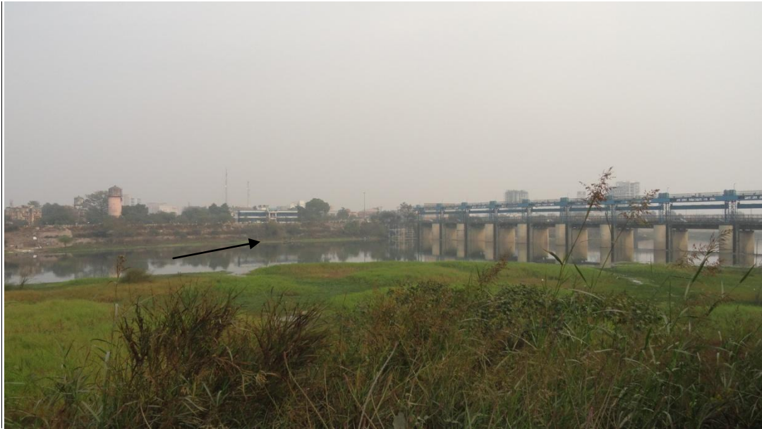
Figure 1a Gomti barrage
