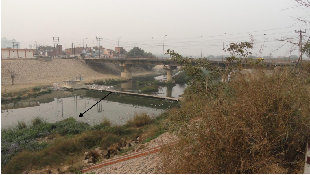
Figure 1e Kukrail nala upstream of its confluence with Gomti river
