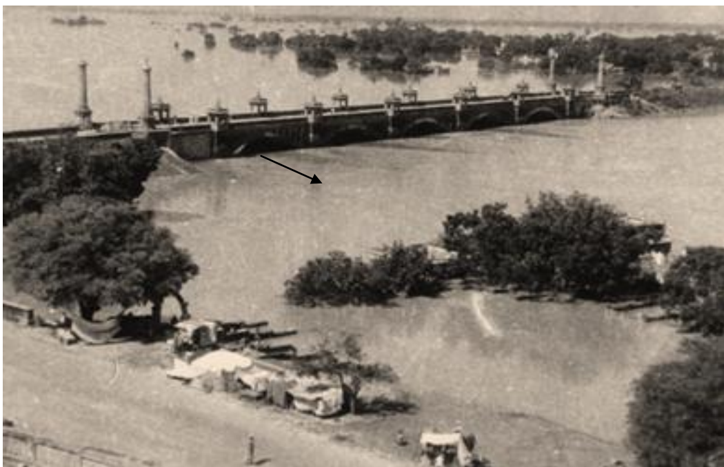
Figure 21 Harding bridge during 1960 flood in Gomti river
