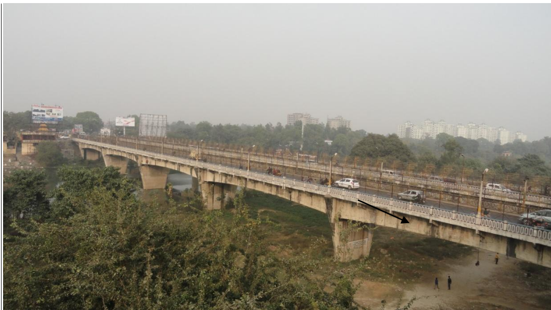
Figure 1b Nishatganj Bridge on river Gomti
